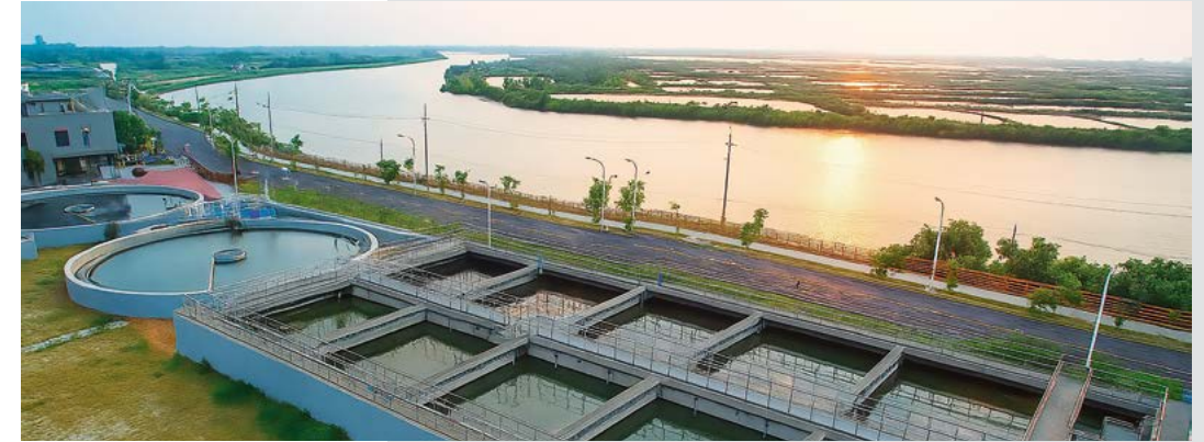
Aerial view of Annan Water Resources Centre
