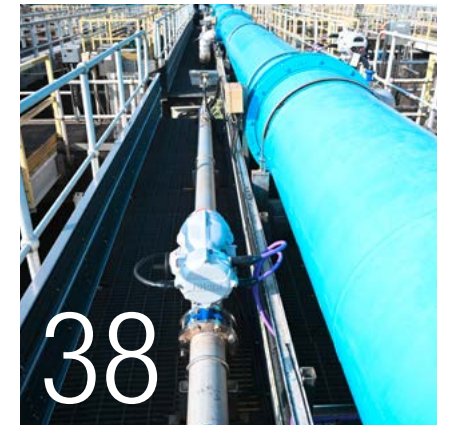
Tai Po Sewage Treatment Works is upgrading its aeration tanks with over 100 AVK Series 76 butterfly valves.
