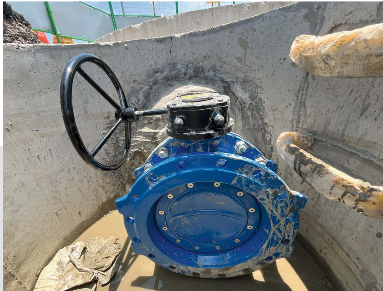
Butterfly valve installed
